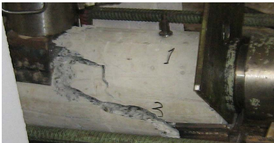
Fig. 2. The destruction of the previous column on ozhatyem old section.
