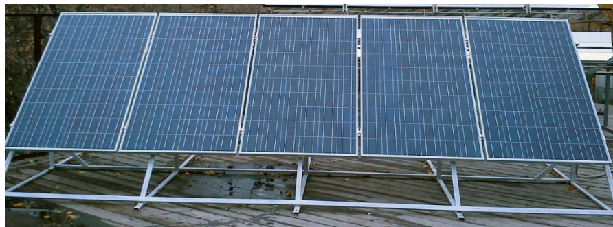
Fig. 6. Solar power plant capacity of 1150 watts
