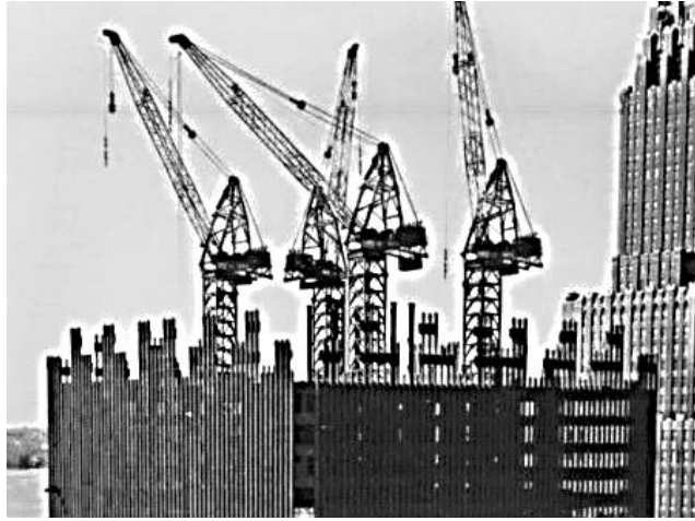
Fig. 3. Tower cranes FavcoSTD 2700.
