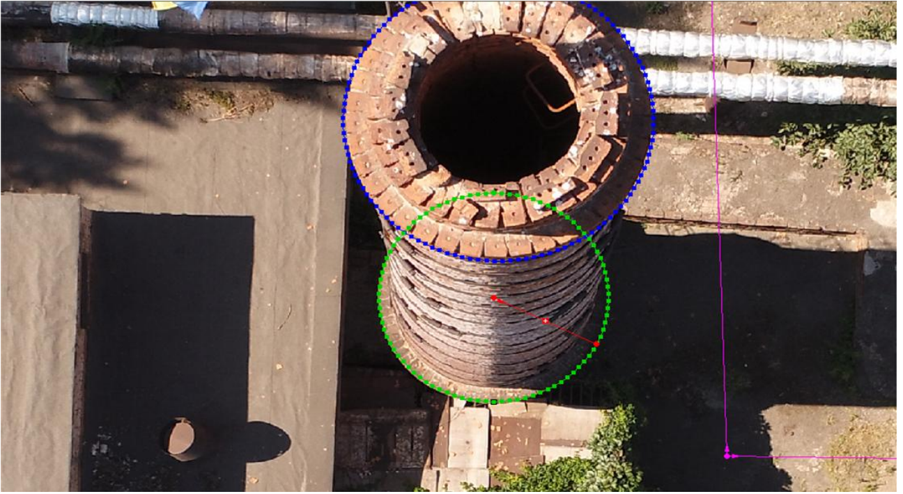
Figure 4. Determination of the center and diameter of the lower cross-section after reconstruction of the missing portion of the chimney ring.
